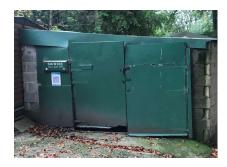
A further pressing project is to refurbish the doors to the garage next to the warden's house. What is needed is simply to make the doors fit the doorframe and make the garage both watertight and neater looking.
